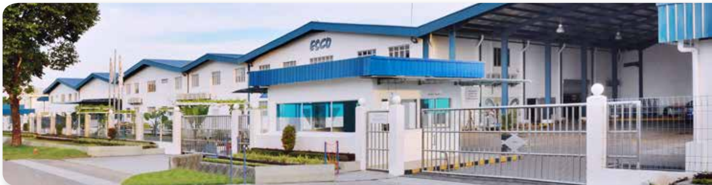
Pictured: Esco's state-of-the-art manufacturing facility
